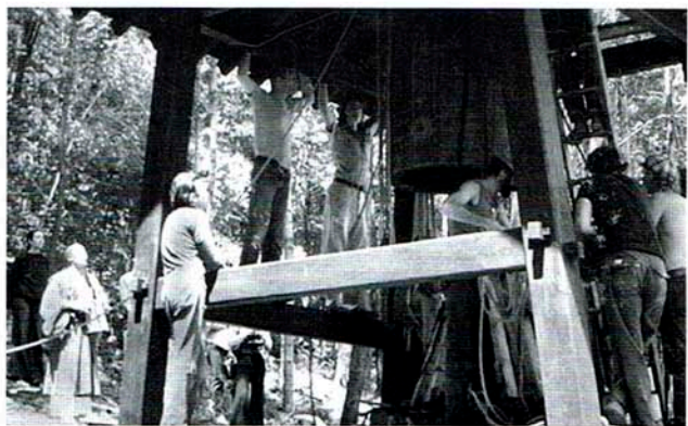
Constructing the Bonsho Tower in 1975
