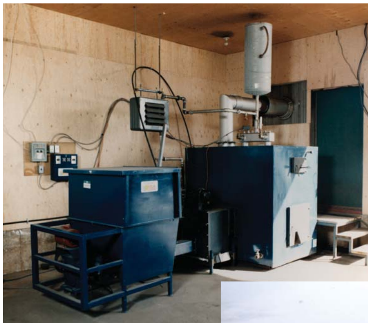
Power Line Pork, Borden, Prince Edward Island Facility Type: Pig farrowing farm System Size: 1 MMBH (two-boiler) Manufacturer: Grove Wood Heat Heating plant is housed in shed on left (lower photo). Fuel is delivered to overhead door and pushed onto shed's floor slab for storage, using tractor. Two side-by-side "Bioblast" systems (like the one in photo at left), located in the same shed, are sized at 45% and 55% of peak load. Each Bioblast consists of a tractor-loaded day bin (shown in foreground), a combustor (middle) and a boiler (rear).
