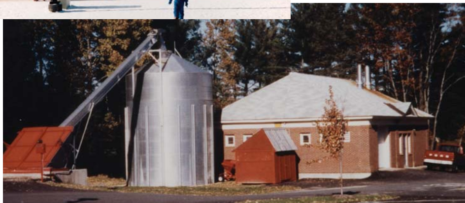
Lyndon Town School, Lyndon, Vermont System Size: 1.2 MMBH Manufacturer: Chiptec Wood Energy Systems This system uses an above-grade metal silo and separate boiler house (which includes garage space). Silo is loaded from a receiving bin (on far left) using an inclined auger.
