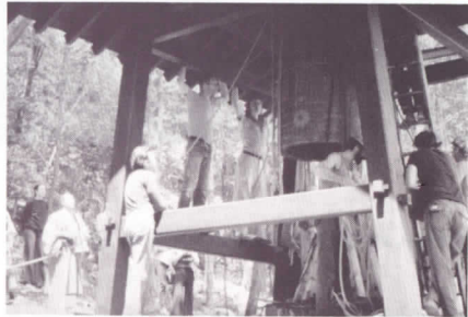
Japanese carpenters at work in the Dharma Hall—May, 1976
