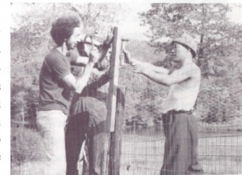
Building the garden fence
